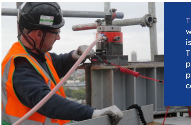
40MM MACALLOY 1030 POST TENSIONING BARS on crane base on Victoria Street, London.
